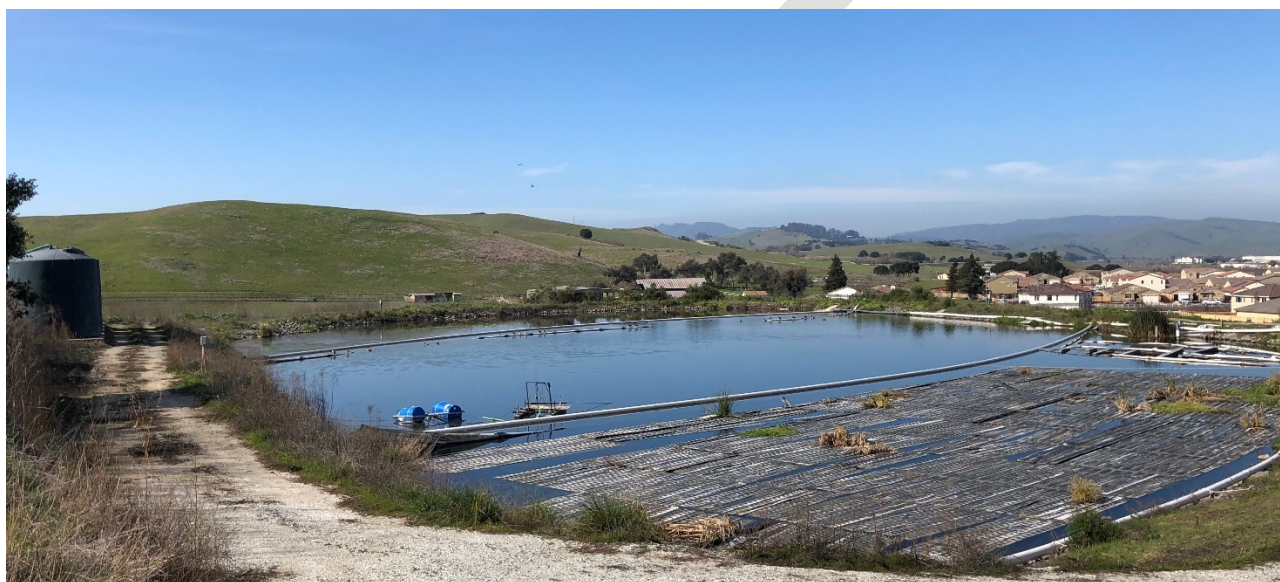
Figure 12 Partition Wall Between Sludge Storage Lagoon and Polishing Pond
