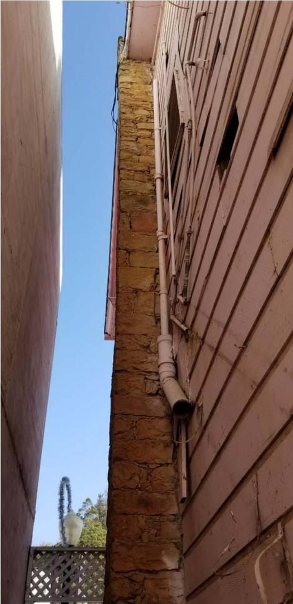
Unbraced unreinforced chimney at exterior.
