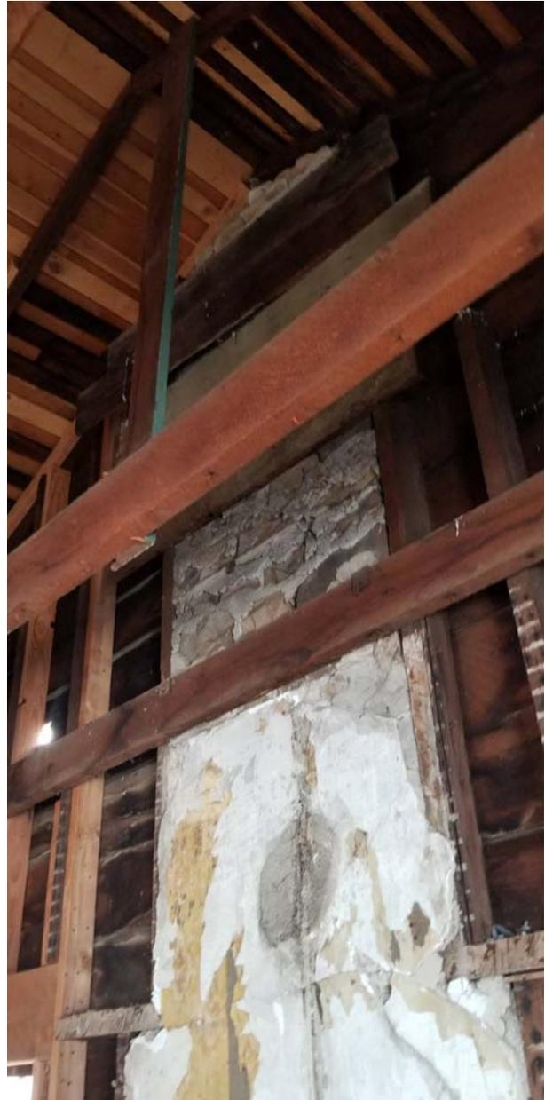
Unbraced unreinforced chimney at interior.
